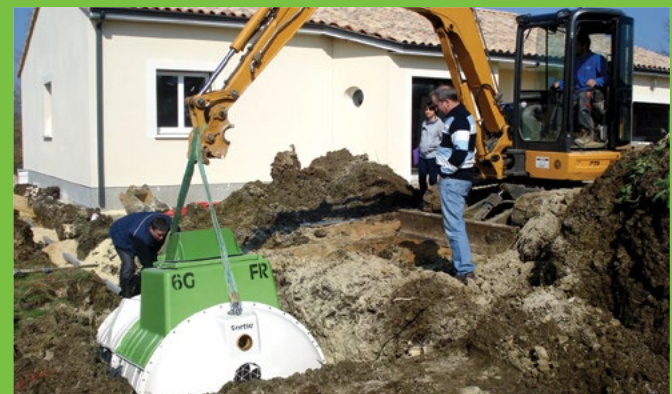
Installation of Tricel Novo FR6
