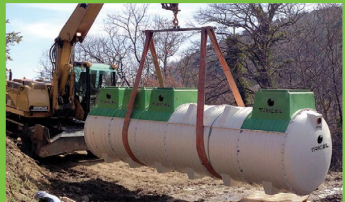
Installation of Tricel Novo FR20
